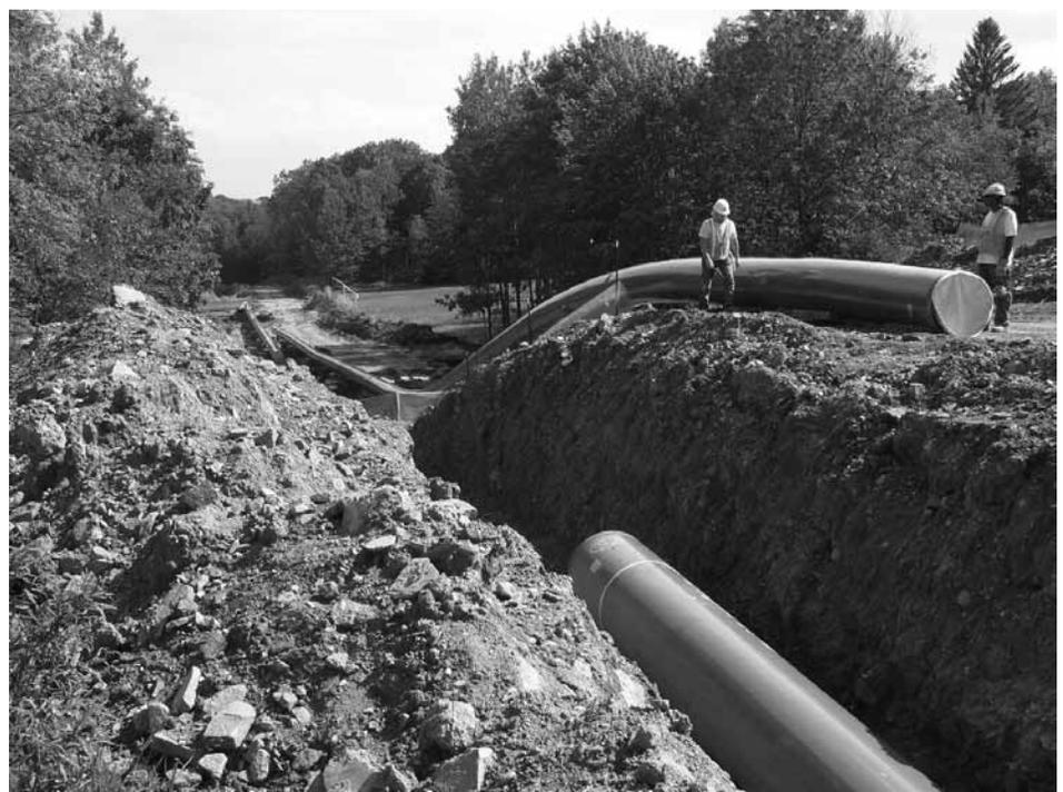
pipeline's path. Coating is applied to the ends of the pipes (the coating applied at a coating mill typically leaves the ends of the pipe clean, so as not to interfere with welding), and the entire coating of the pipe is inspected to ensure that it is free from defects.
