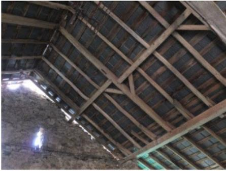
*The Ferry stone to the peak Standard barn at the southwest end of Centennial Road was built circa 1820. Barn has Principal Rafter System where principals are much larger than common rafters at either side of the Principals. Staggered purlin plates intercept the Principals.*
