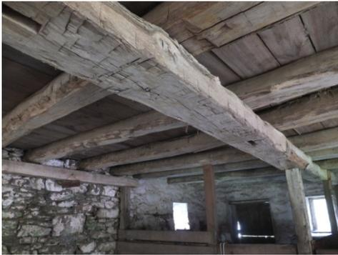
*The Murphy stone barn off Longswamp Road in its basement has its original barn length summer beam seen from upper left of photo to near lower right corner of photo. Above the summer is a series of transverse ceiling joists. Joists in turn support the upper floor level.*
