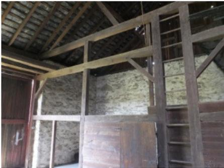
*The Murphy stone to eaves level Standard barn on the south side of Longswamp Road was built circa 1850. Transverse bent on upper floor level has posts, built-in ladder and braces with partial barn width ties. At top of bent is upper tie than joins to wall plates.*
