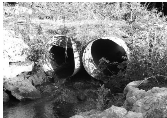
Photo shows the two metal pipes to be removed.
